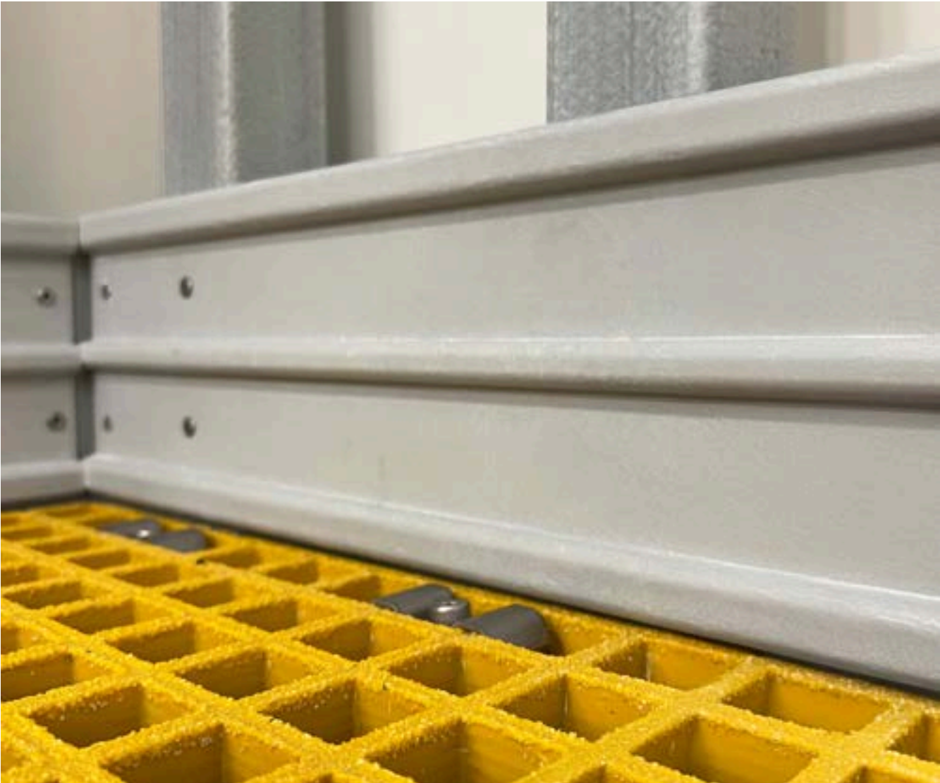
Kick plate for fiberglass railing systems.
