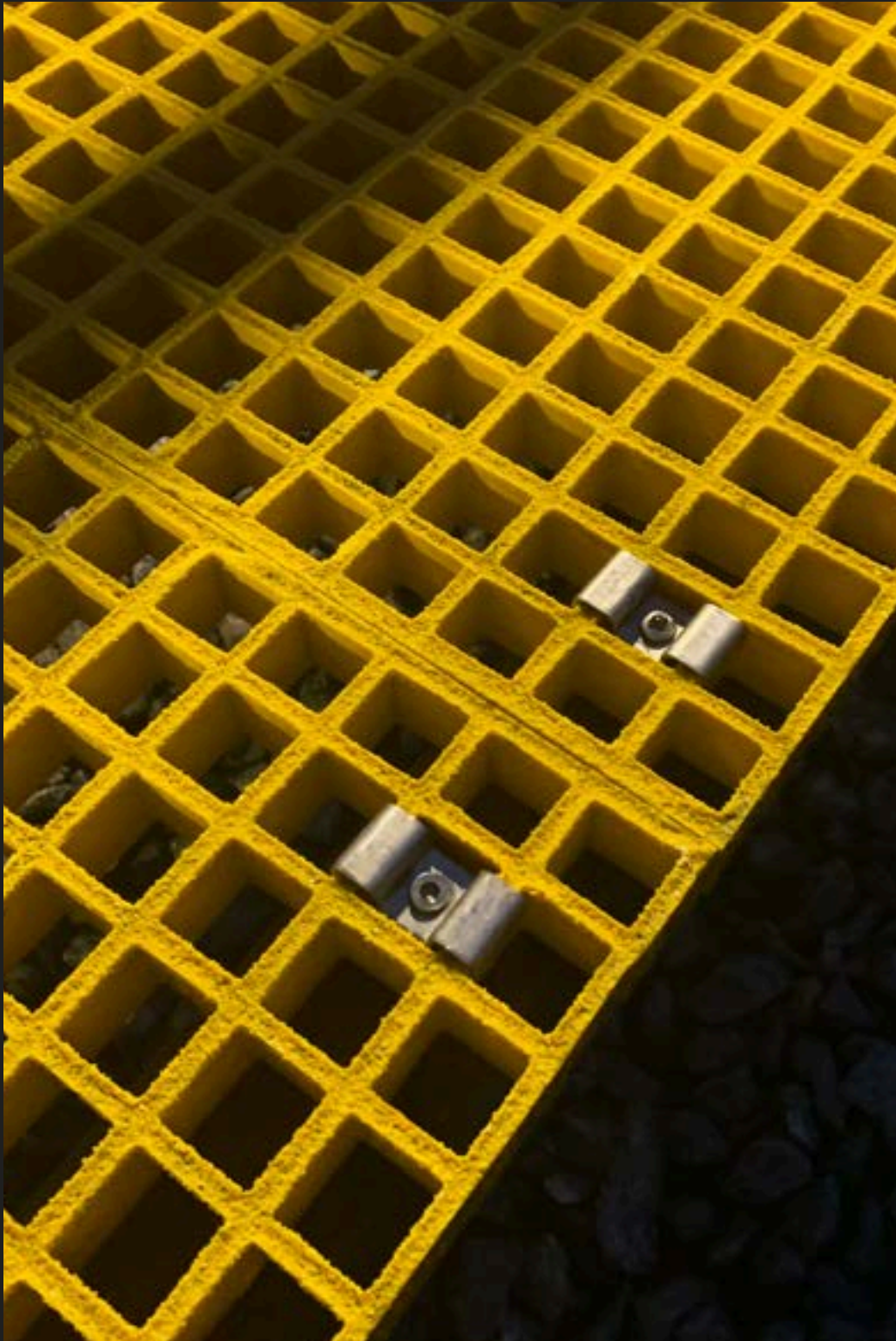
ISO 30, sanded. MK-clips, stainless steel.
